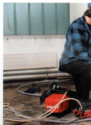
Top coring efficiency in plumbing
